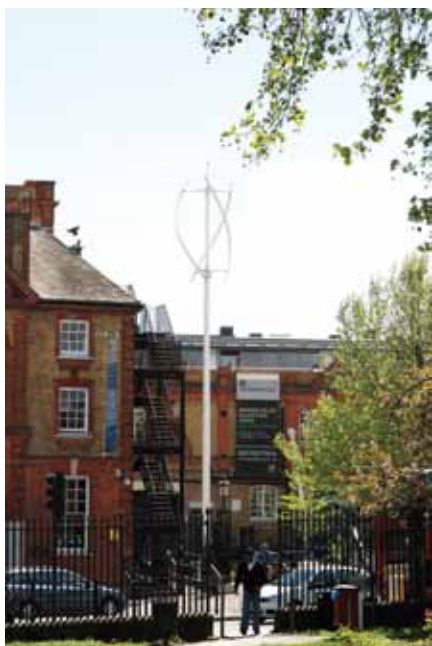
Wind turbines are often found as decoration on commercial buildings to make them appear to be more sustainable than they really are. However the increased surface friction due to the buildings in urban environments means that the power that can be extracted from the wind is only a fraction of that possible in open countryside.
