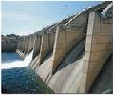
Figure 1: Construction of a major dam
