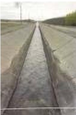
**Figure 1:** Open channel drainage system
