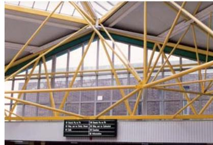
**Figure 5:** *Space Frame Roof Structure*
