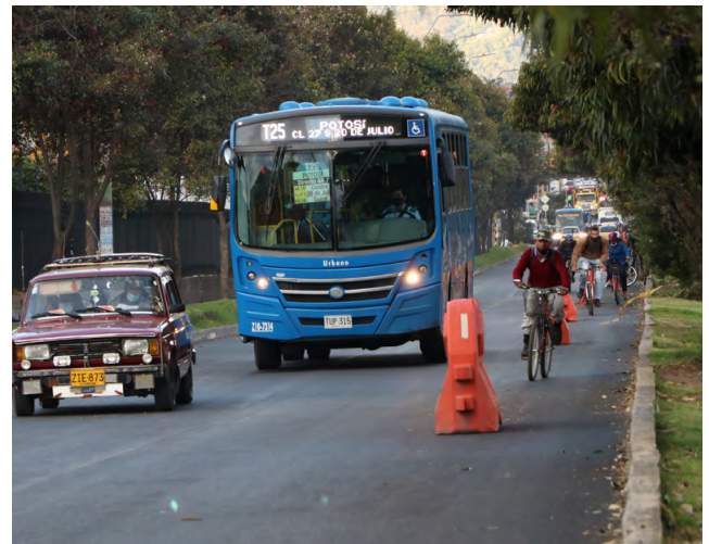
b) Temporary bike path
