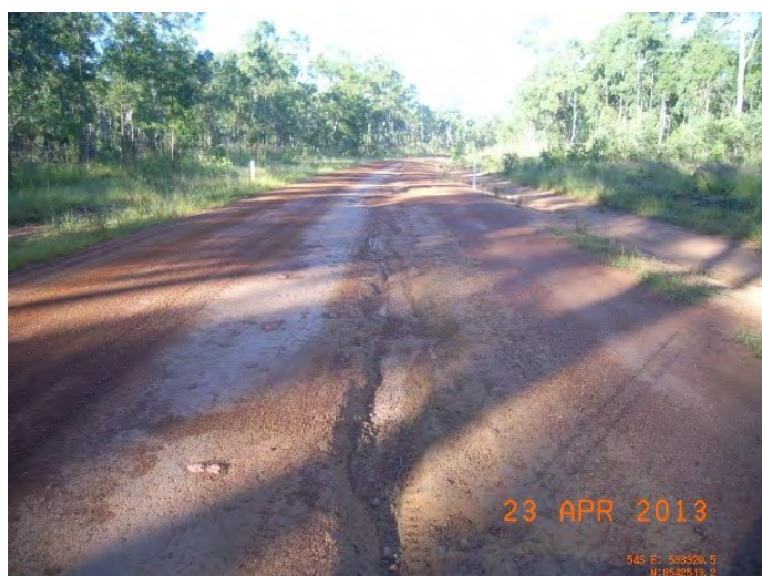
Figure 4: Arukun Access Road (the only road link to and from the Arukun community). Left: Gravel road that was damaged in 2010, 2011, 2012, and 2013. Right: Bitumen seal instated in 2013 along a 10 km vulnerable section. This has since withstood impacts of eight natural hazard events (photos courtesy of the QRA).
