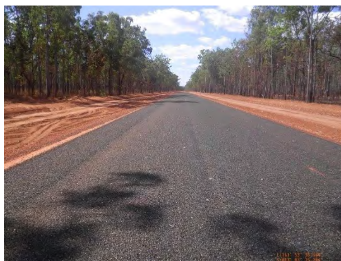
Figure 4: Arukun Access Road (the only road link to and from the Arukun community). Left: Gravel road that was damaged in 2010, 2011, 2012, and 2013. Right: Bitumen seal instated in 2013 along a 10 km vulnerable section. This has since withstood impacts of eight natural hazard events (photos courtesy of the QRA).
