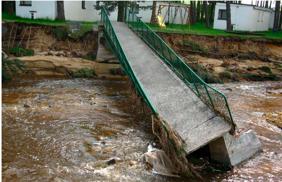
Damage caused to a bridge by heavy rain and flooding
