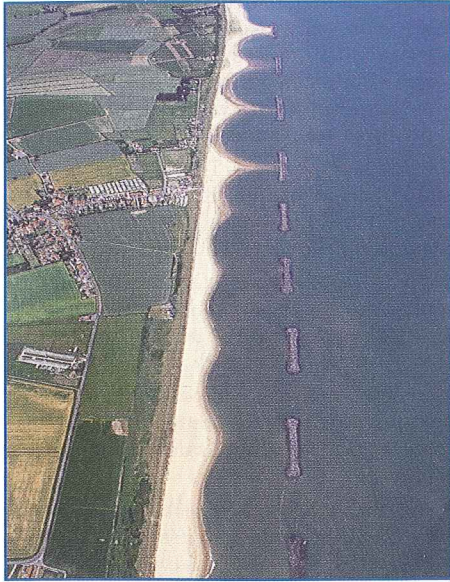
Breakwater scheme at Sea Palling, Norfolk (Courtesy of Mike Page)
