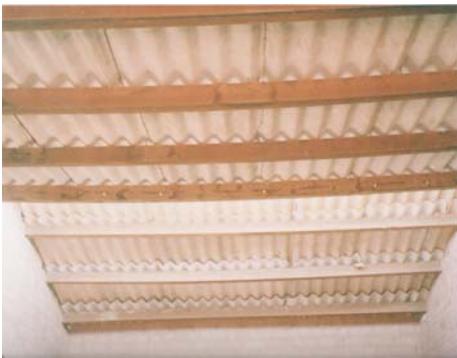
Figure 4 – A school building constructed with CSSB walls and fibre-reinforced cement roofs.
