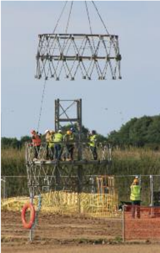
Figure 14: Constructionarium: Scale Swiss Re Tower
