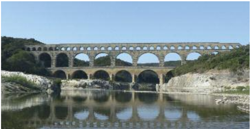
Figure 2: Pont du Gard, France
