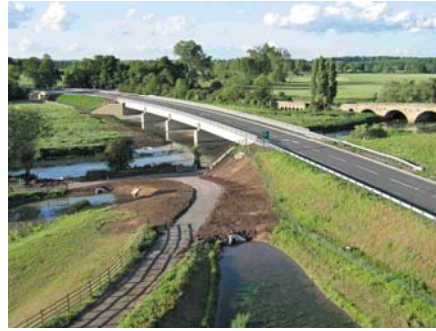
Figure 2 Construction of a highway
