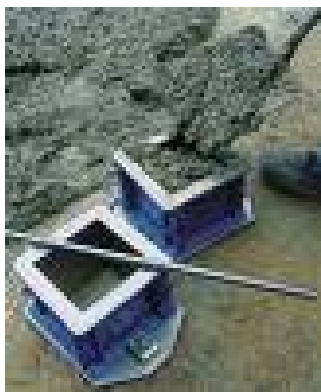
Figure 1: Moulds for making cubes
