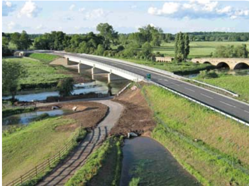
Figure 3: Road curving over a river
