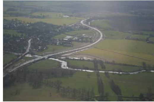
Figure 2 Road alignment as seen from the air
