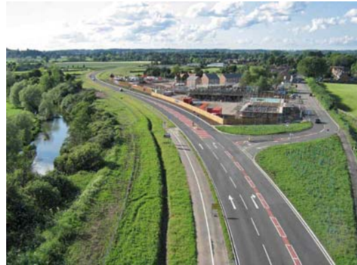
Figure 4 Road with junctions after construction
